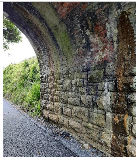
Masonry arch bridge along the greenway
