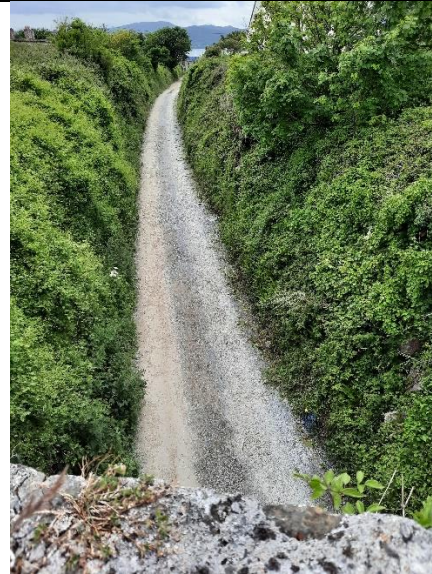
View of the greenway from a masonry bridge
